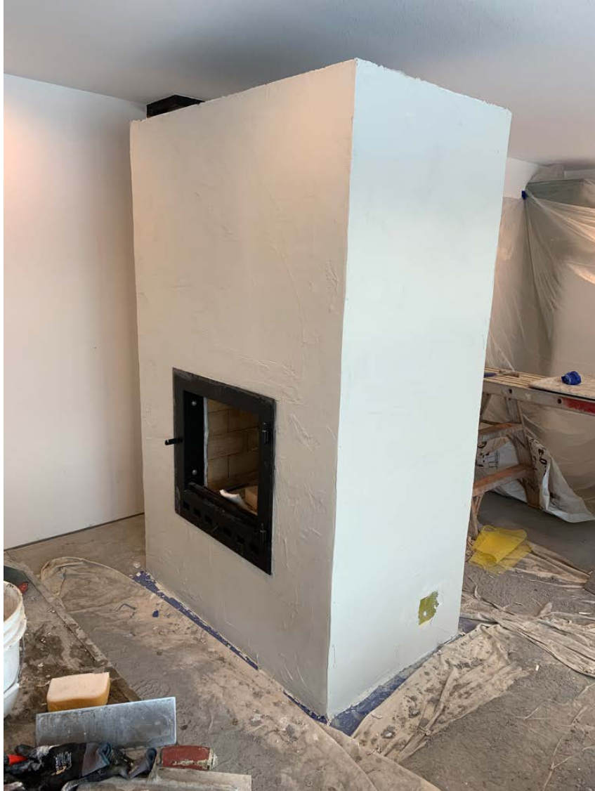
Second coat of thin set is applied to all 4 sides of the heater.
